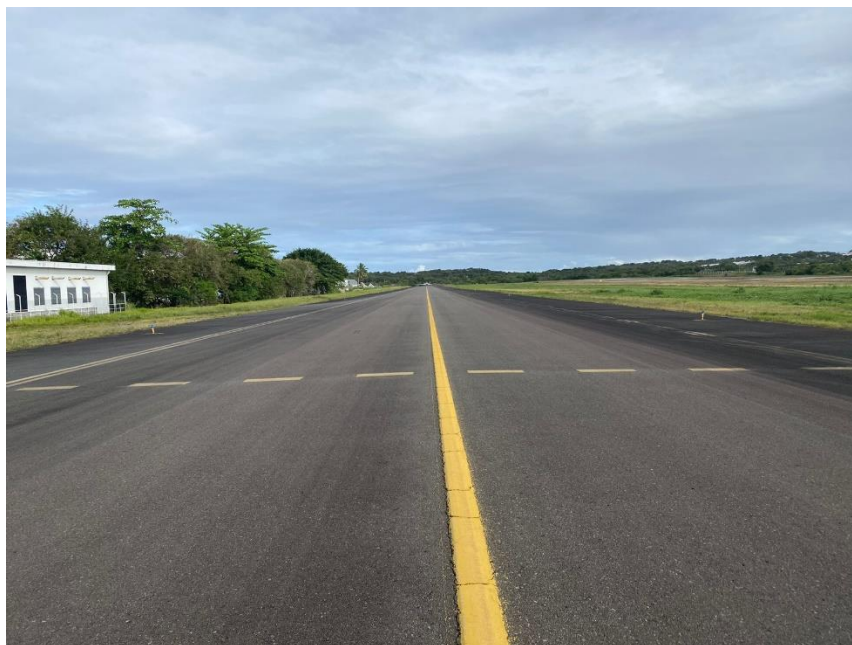
Figura 4 – Pista de Taxiway Mike
